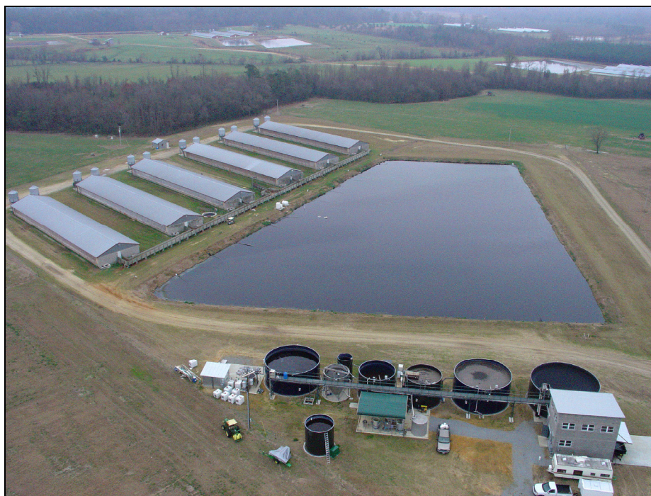
Figure 1. Full-scale wastewater treatment system (project activity) that replaced the anaerobic swine lagoon (background), Duplin County, North Carolina
