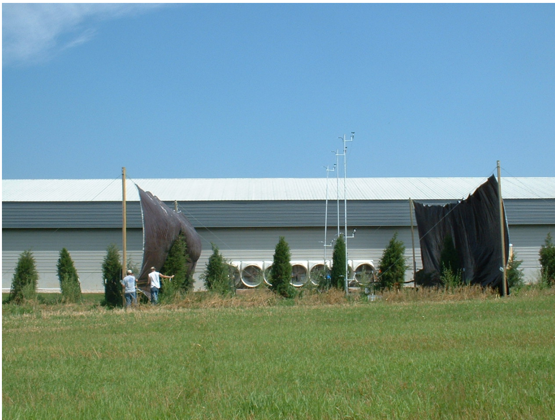
Figure 3. PMT set-up with sampling diversion curtains extended
