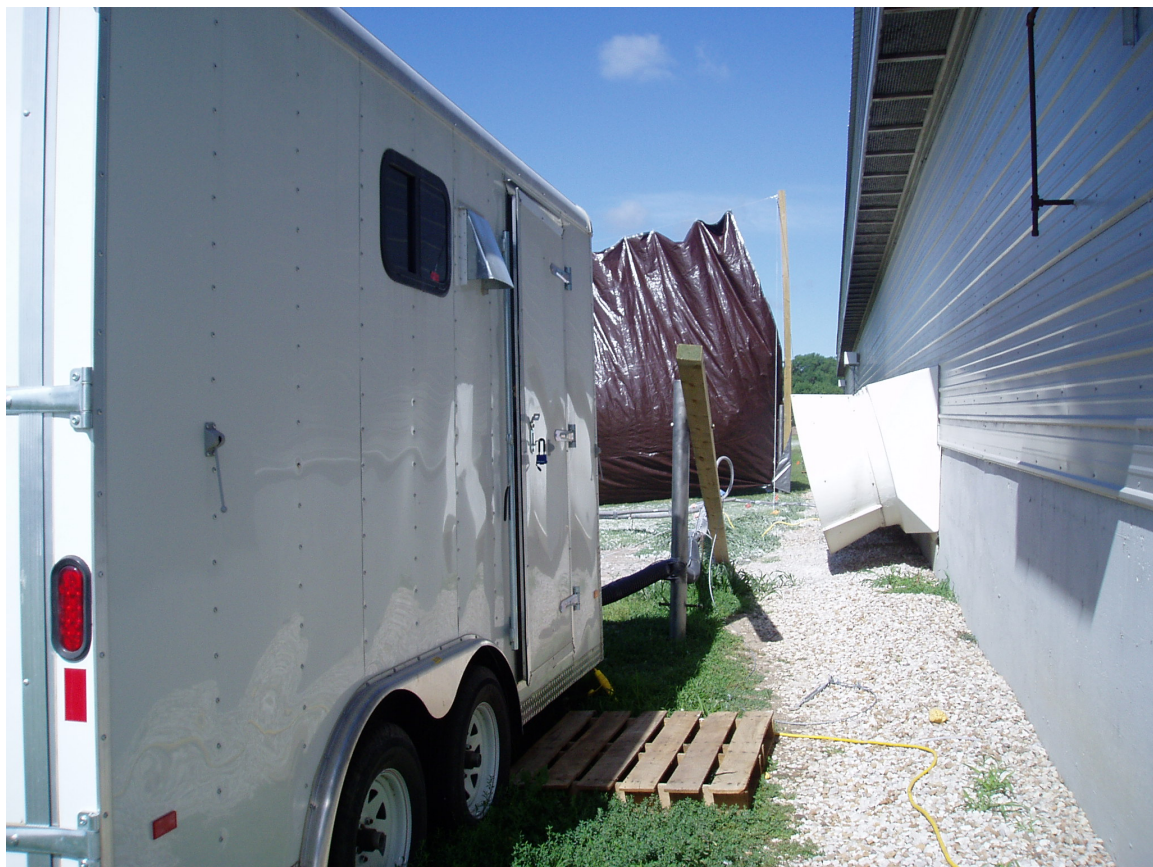
Figure 2. MEL shown installed on-site
